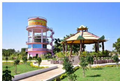
Overhead Water Tank
