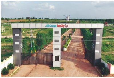
Entrance Arch with Compound Wall
